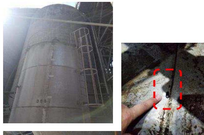
Oil leakage
