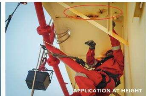
ANGLE BAR CORROSION
