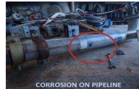
CORROSION ON PIPELINE
